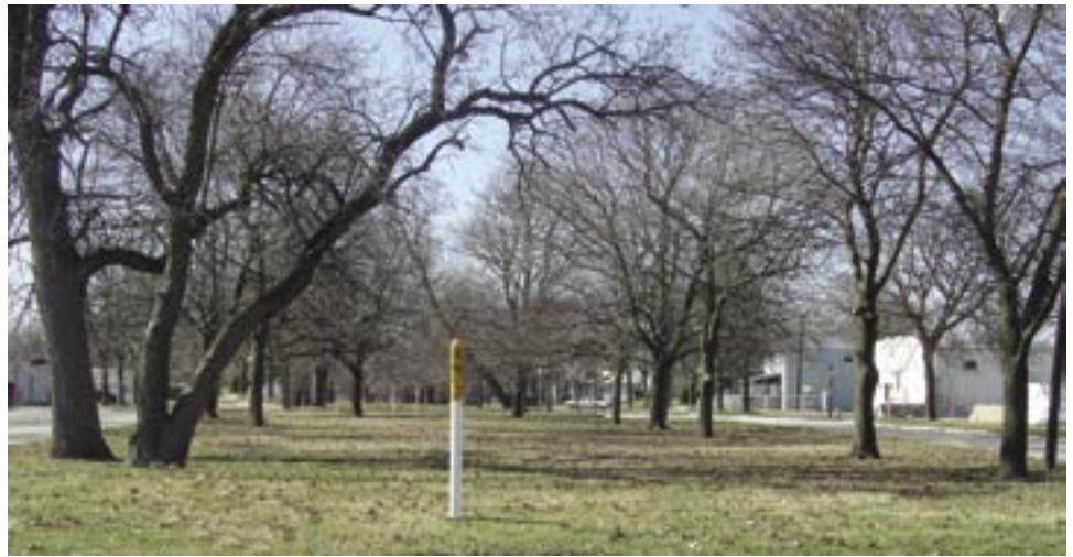
Keeping pipeline right-of-ways clear is critical to safety.
